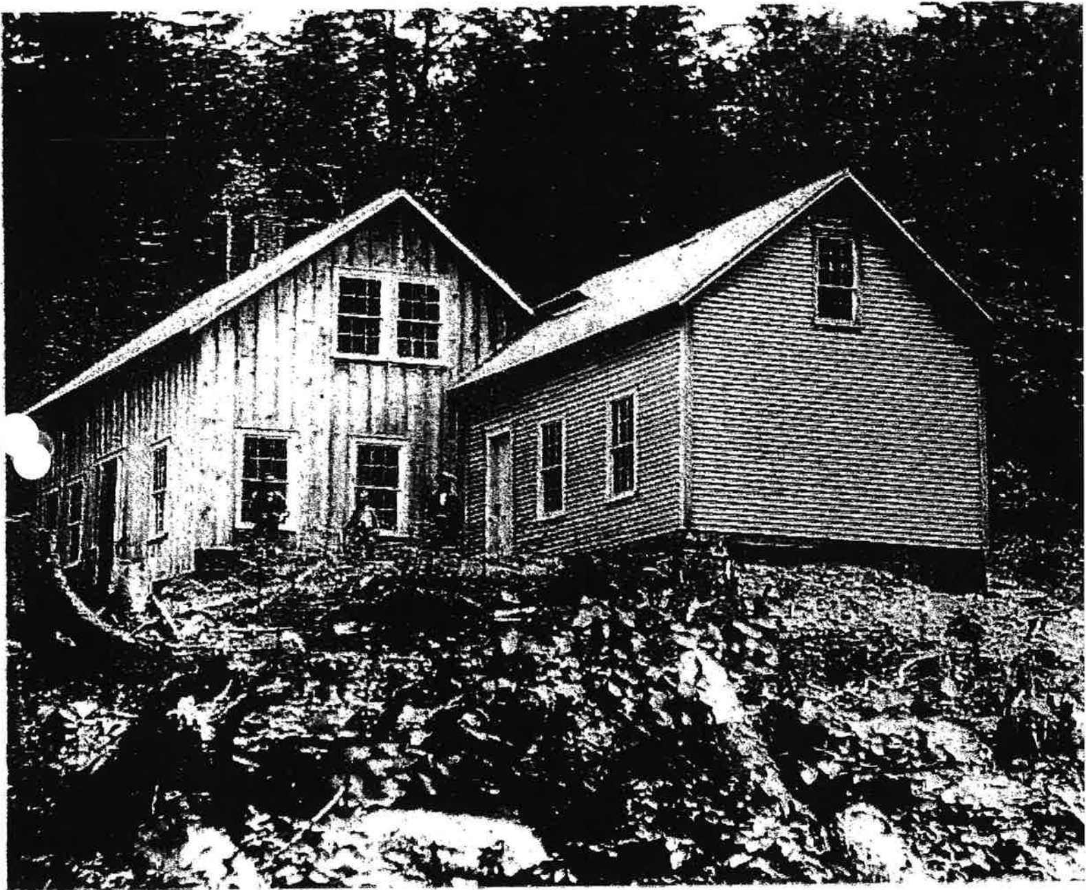
HALFWAY HOUSE c.1867
