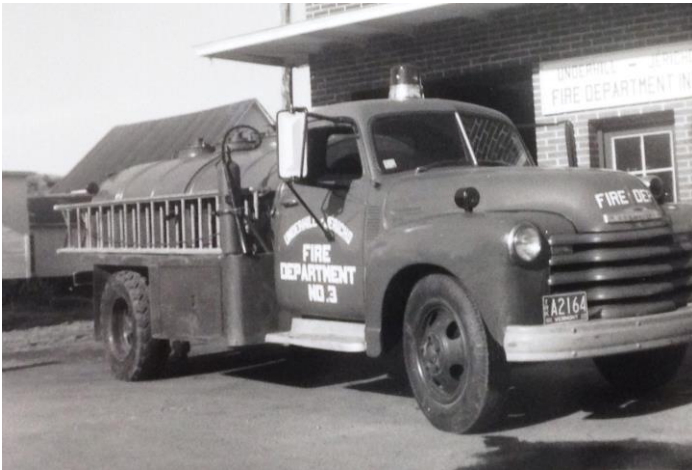
1952 Chevrolet 850 gallon converted fuel oil truck to tanker
