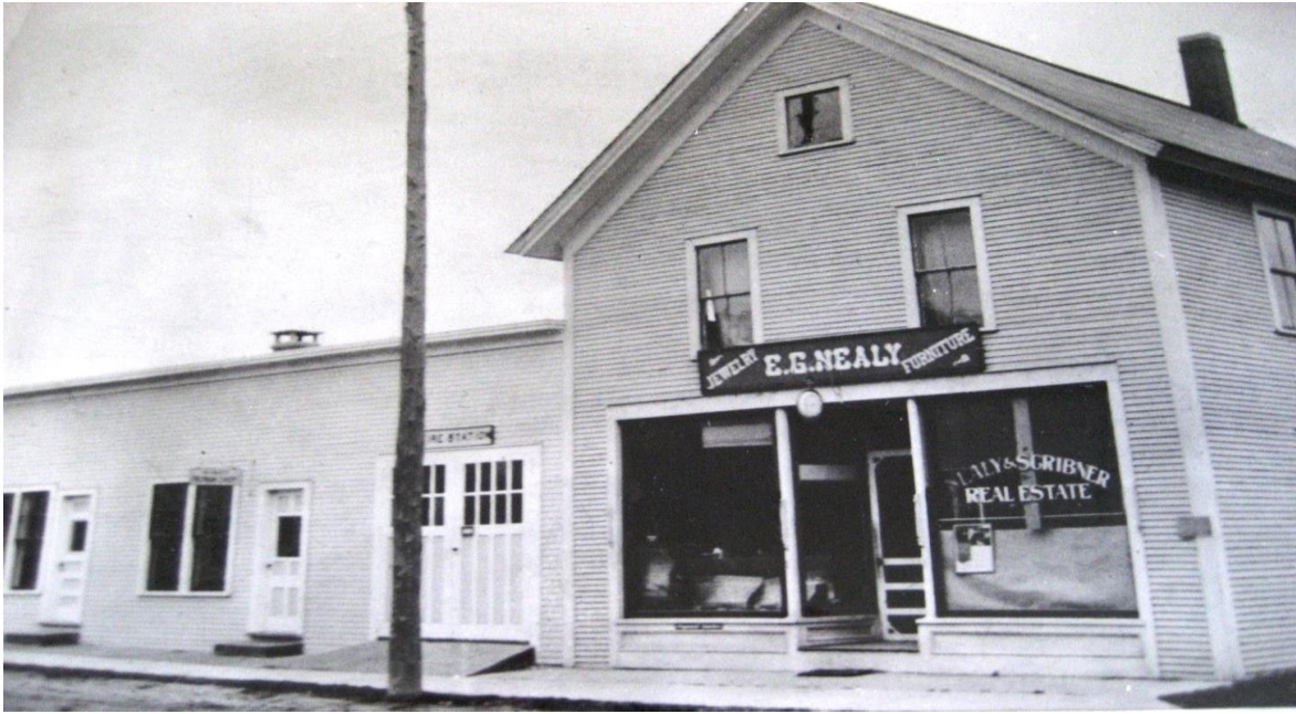
The Underhill Fire Station located on Park Street
