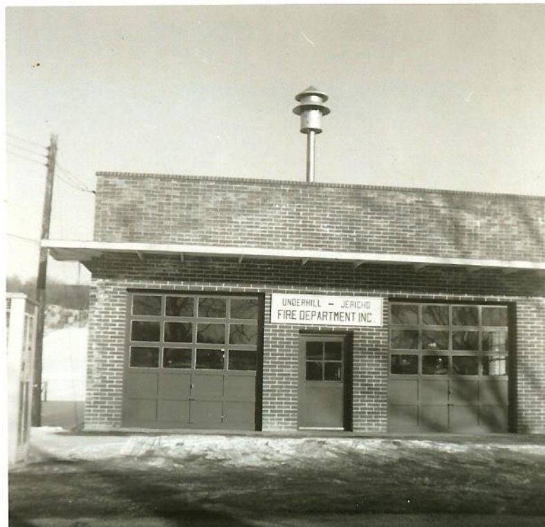
New brick Fire Station built with mostly volunteer labor 1952
