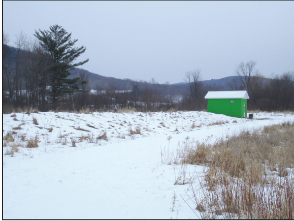
Figure 3. Well Point Field and Pump House
