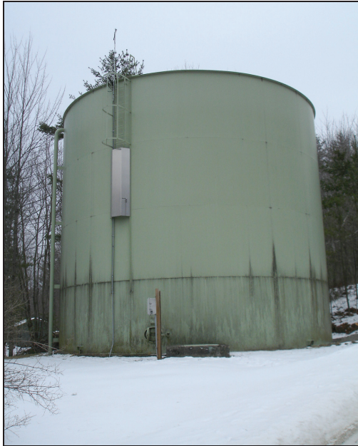
Figure 2. Maple Ridge Water Storage Tank
