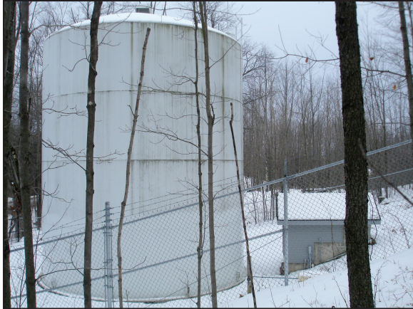
Figure 9. Poker Hill Storage Tank
