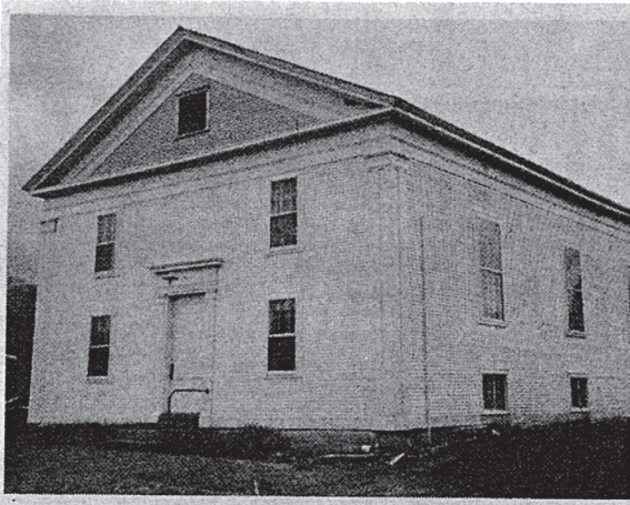
UNDERHILL TOWN HALL , Underhill Center — A frame building built in the mid-1850s in Greek Revival style. Underhill can be proud of the heroic effort put forth in recent months to render this old building useful for contemporary community needs. The citizens organized as the Underhill Historical Society and found a variety of ways to raise the necessary money. The basement has been done over to house the town library and the town clerk's office, with a fireproof walk-in vault and new carpeting. Upstairs the main assembly room has been redecorated for town meetings. Electric heat has been provided throughout the building, and the exterior has been painted.
